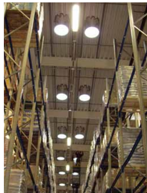
magazzino, Lightway® Silver 600
